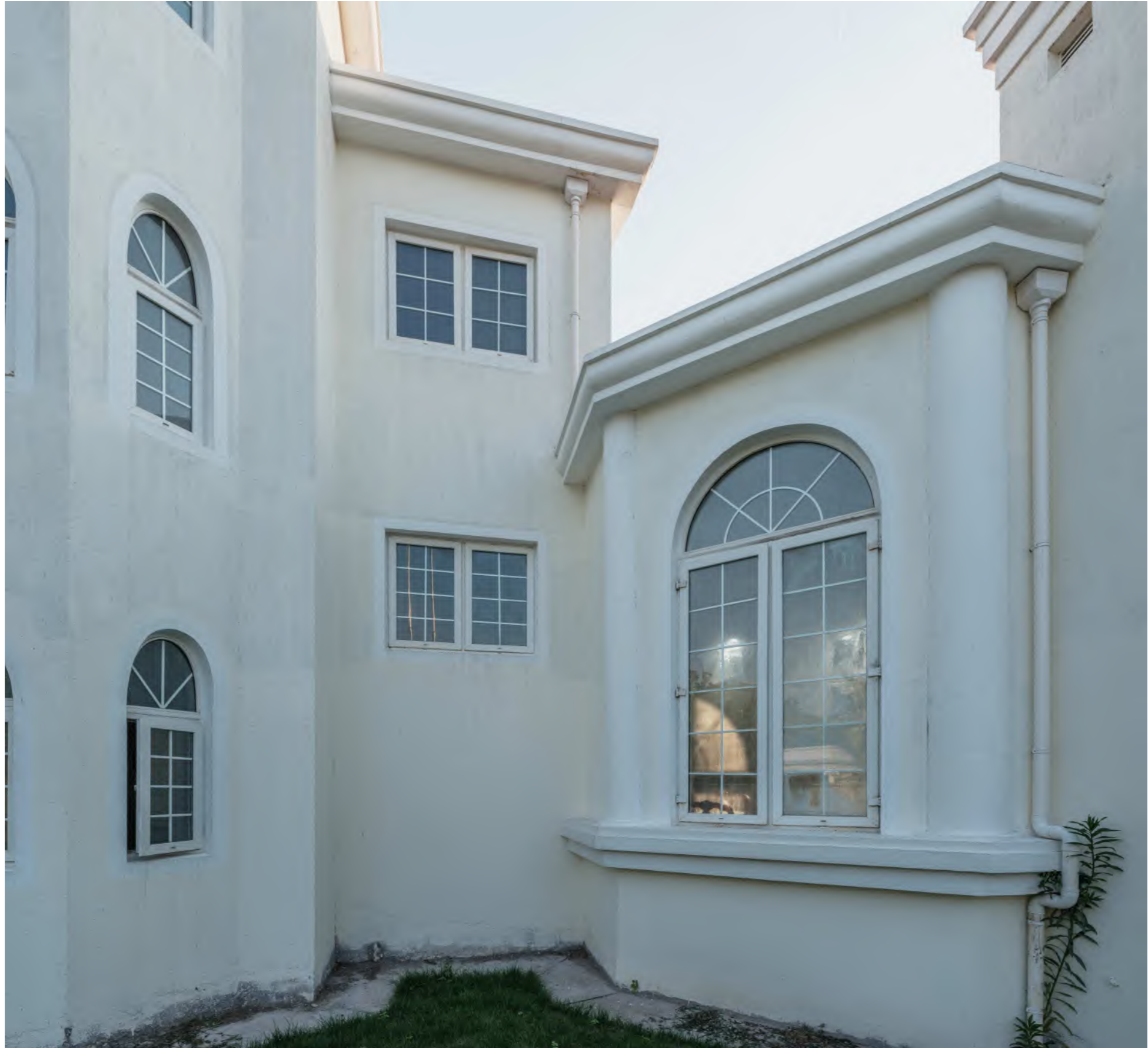
outside building - 整栋外立面
